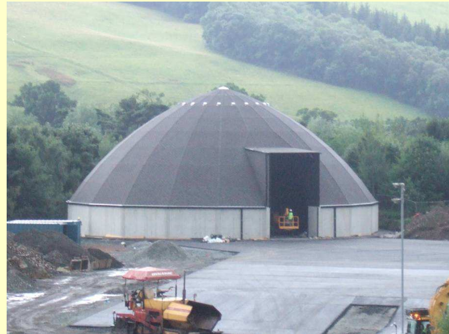
Newest salt storage facility at Eshiels Depot Peebles with a holding capacity of 5000 tonnes
